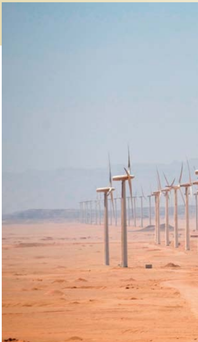
The Zafarana wind farm in Egypt saves the country 332,000 tons of fuel a year, and reduces annual carbon emissions by approximately 834,000 tons © New & Renewable Energy Authority, NREA, Egypt
