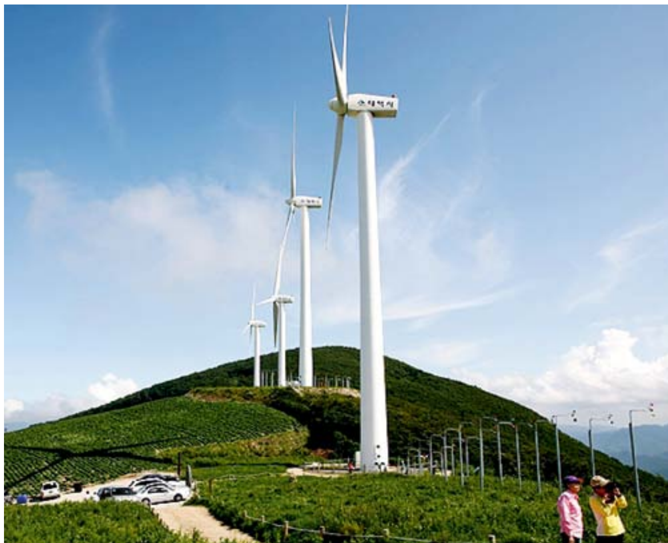
18 MW Taebaek wind farm in Kangwon Province. Hyundai 2MW x 4WTG's & Hyosung 2 MW x 5 WTC's, commissioned in May 2012 © KWEIA
