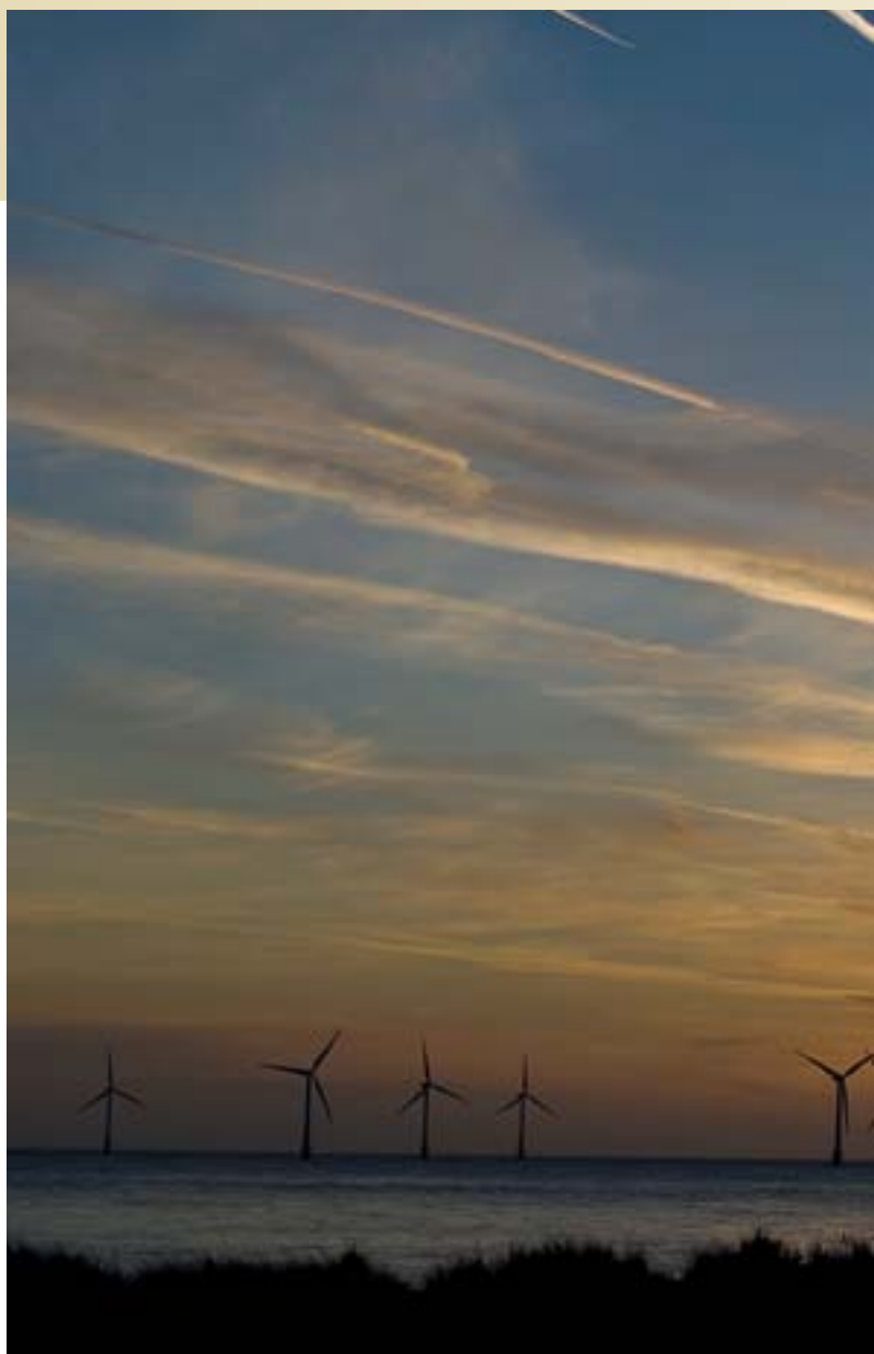
Scroby Sands Offshore Wind Farm, Great Yarmouth, UK © RenewableUK
