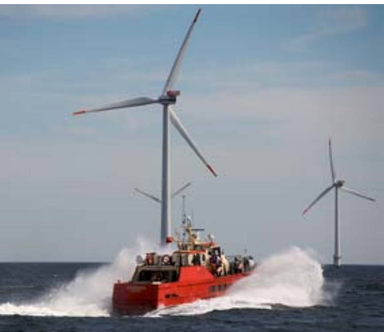
Horns Rev II wind farm, Denmark © Wind Power Works
