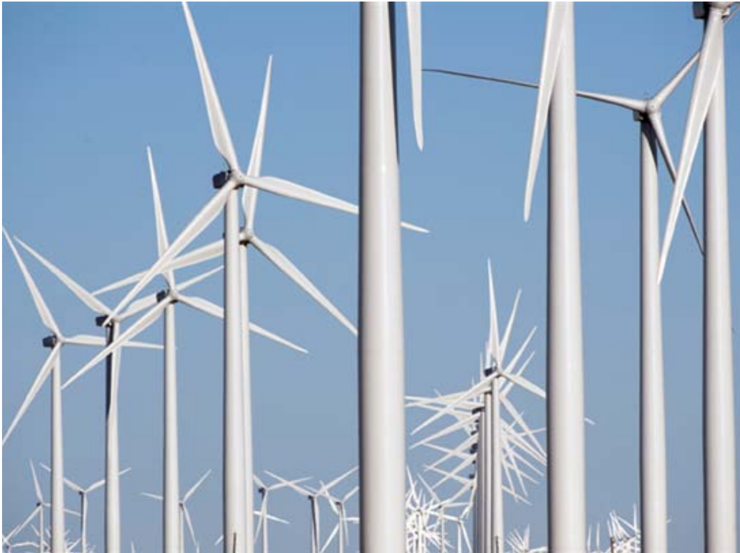
Horse Hollow wind farm, Texas, US © Wind Power Works
