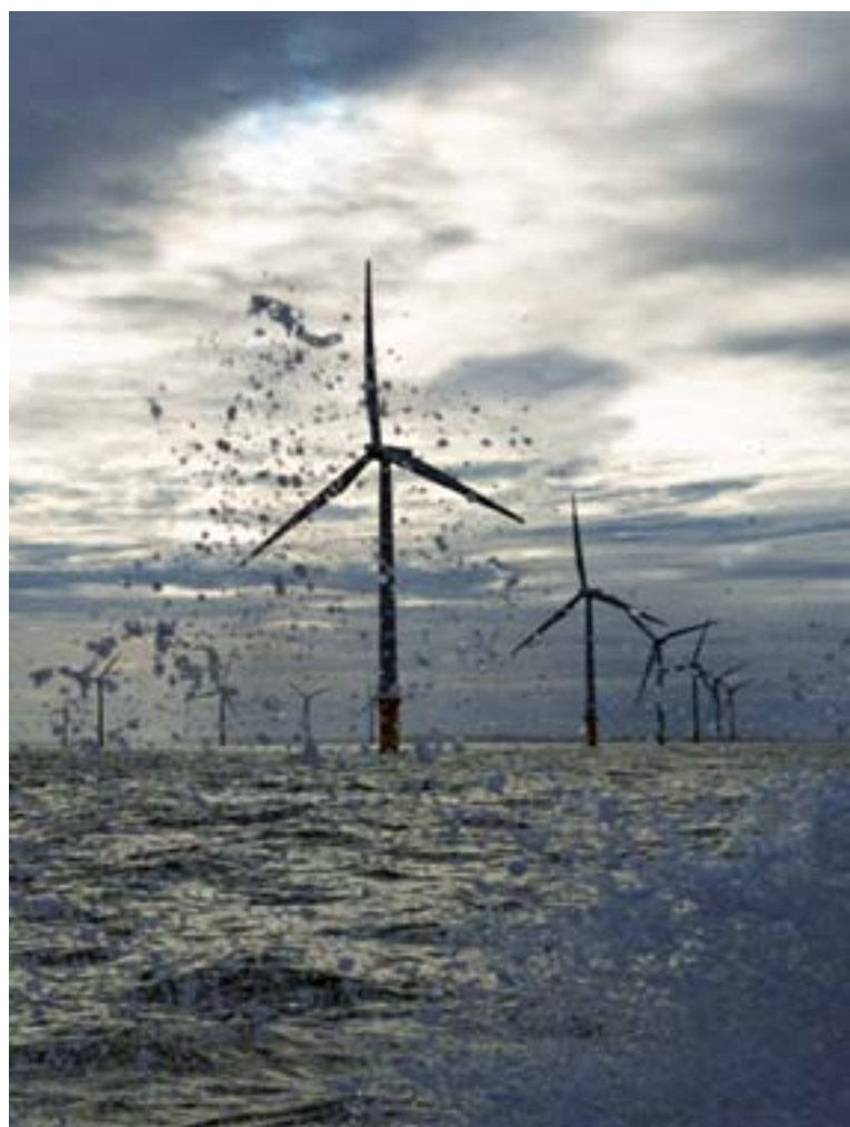
Burbo Bank wind farm, Liverpool Bay, UK © Wind Power Works
