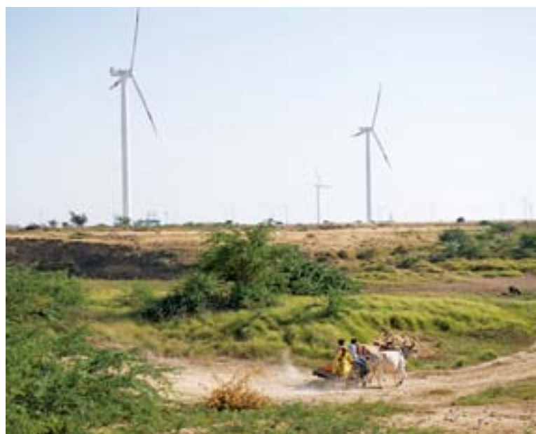
Kutch wind farm, Gujarat © Wind Power Works
