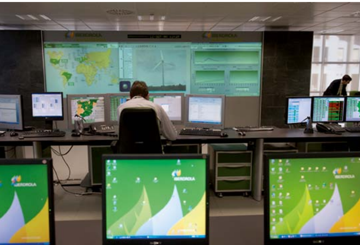
Iberdrola control center, Spain © Wind Power Works
