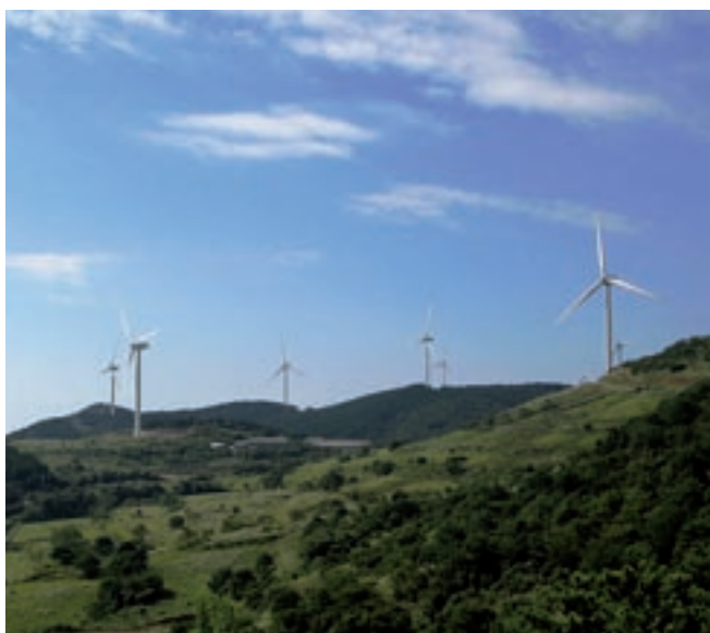
Nagashima wind farm (Photo: Japanese Wind Energy Association)
