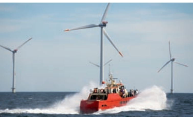
Denmark, Horns Rev II, North Sea (Photo: Wind Power Works)
