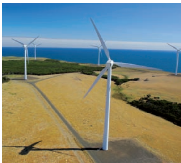
Woolnorth wind farm (Photo: Roaring 40s)
