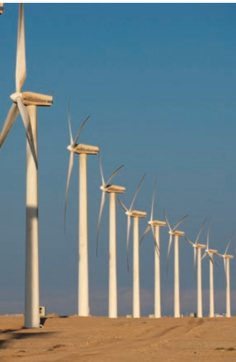
Zafarana wind farm (Photo: Wind Power Works)
