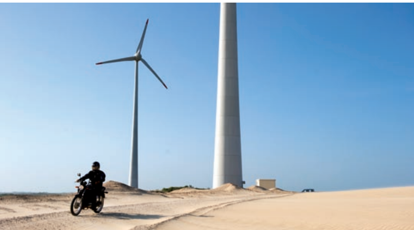
Rio do Fogo wind farm (Photo: Wind Power Works)
