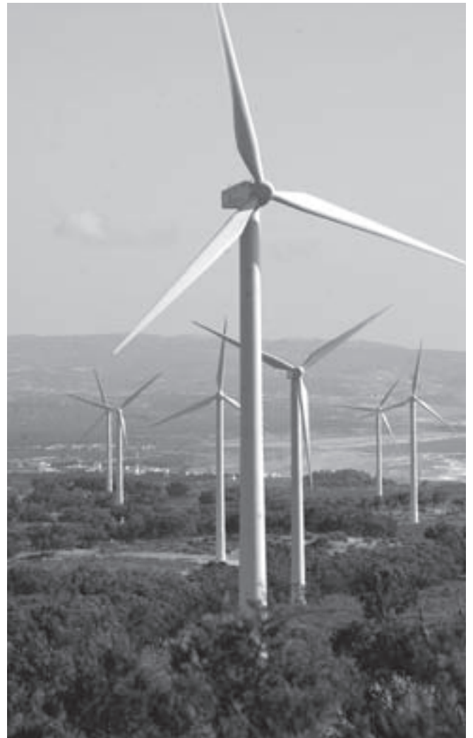
Amogdoul wind farm, Morocco
