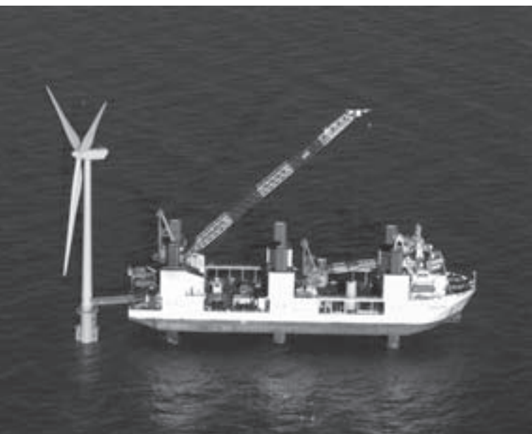
Barrow wind farm, UK
