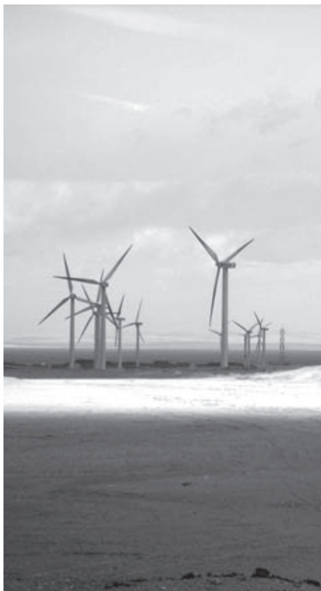
Zafarana wind farm, Egypt
