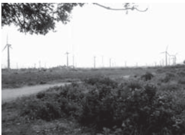
Wind farm located near the Coimbatore Area of Tamikl Nadu
