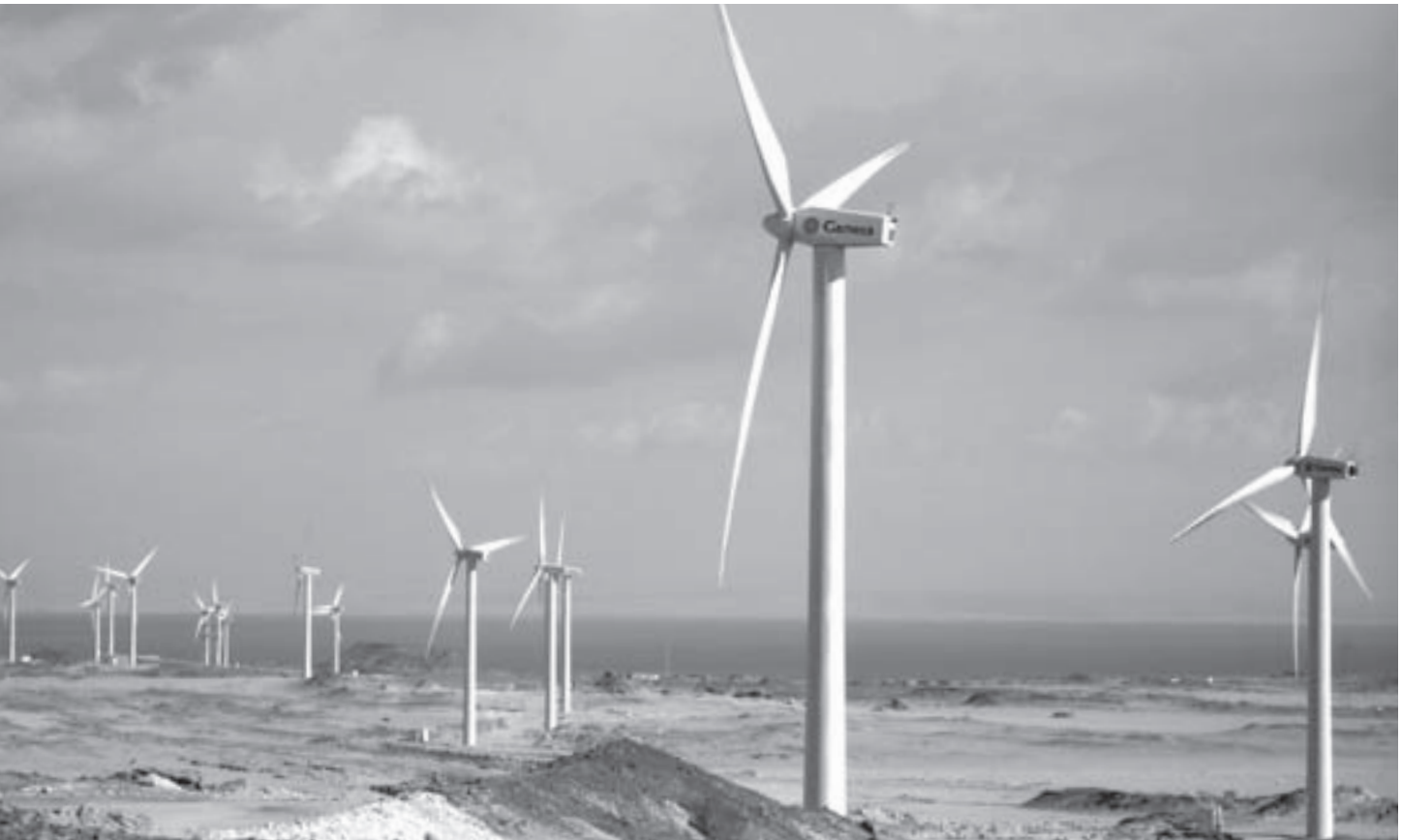
Zafarana wind farm, Egypt
