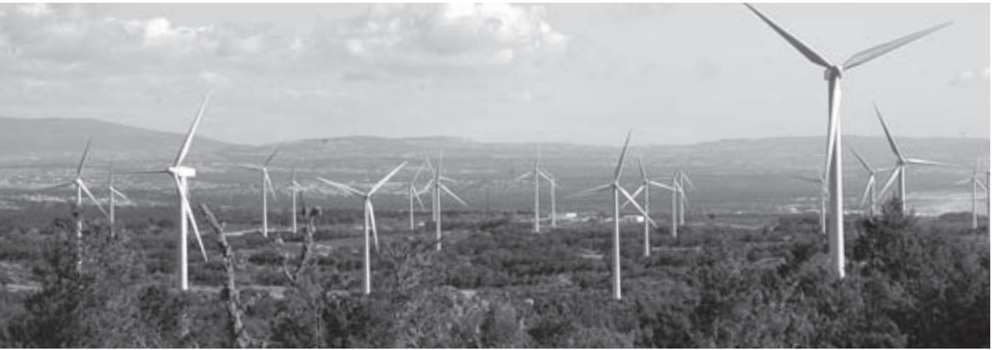
Amogdoul wind farm, Morocco
