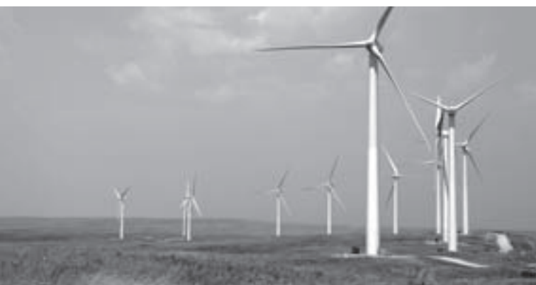
Soderglen wind farm, Southern Alberta, Canada
