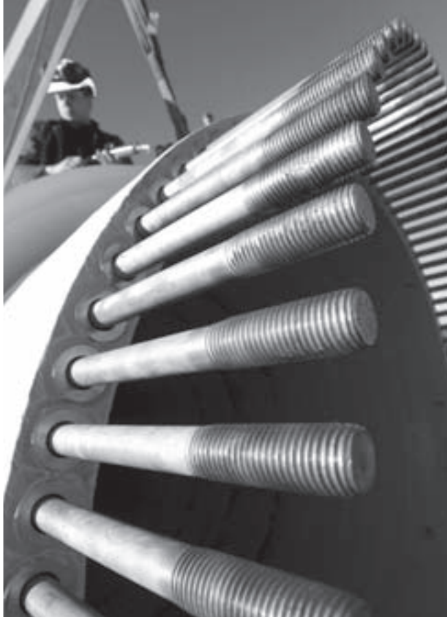
Construction site Vestas, Porep, Germany
