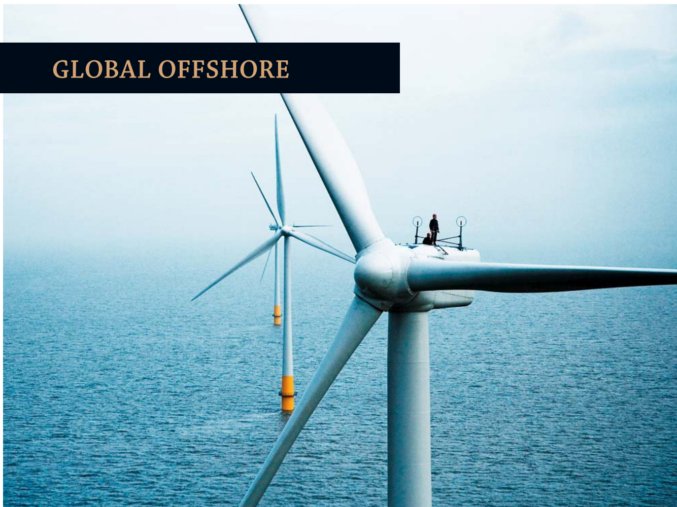
Offshore service © Vestas-MHI
