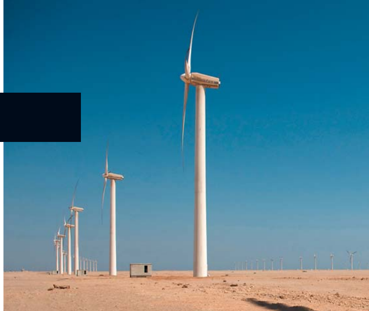
200 MW El Zayt Wind Farm (under construction), Egypt © RCREEE
