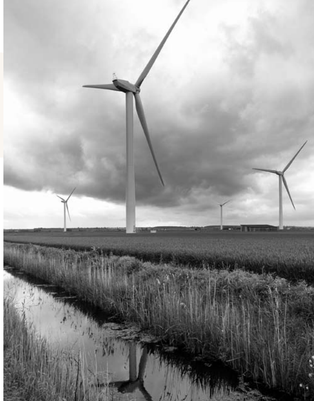
Red Tile wind farm
