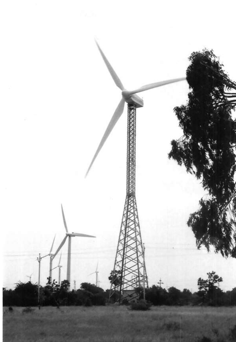
Wind farm located near the Coimbatore Area of Tamil Nadu
