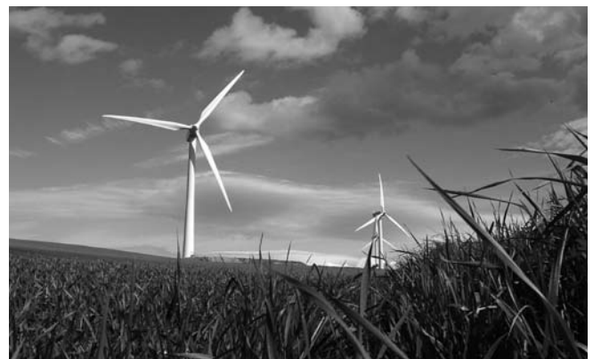
Whitelee wind farm © Scottish Power
