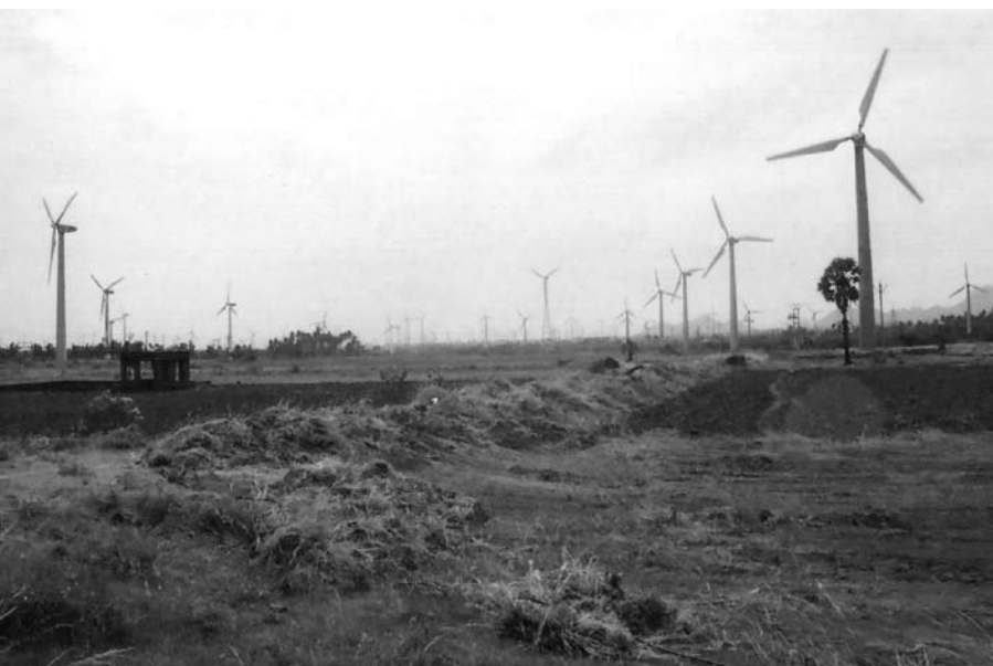
Wind farm located near the Coimbatore Area of Tamil Nadu
