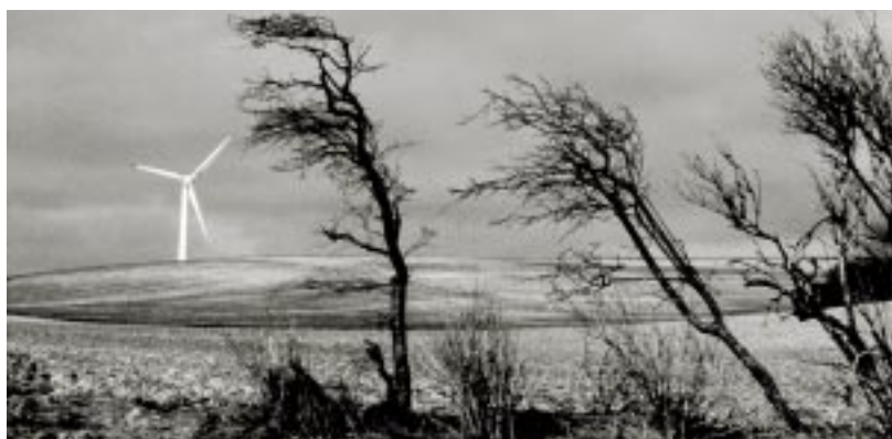
Wind farm, France
