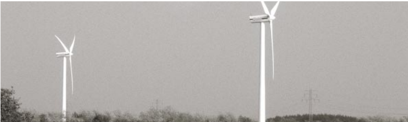
Wind turbines in Denmark
