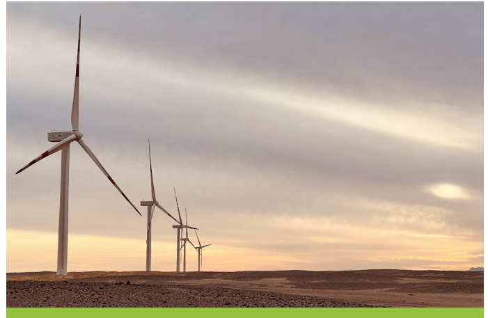
Photo: Courtesy of West Bakr wind farm
